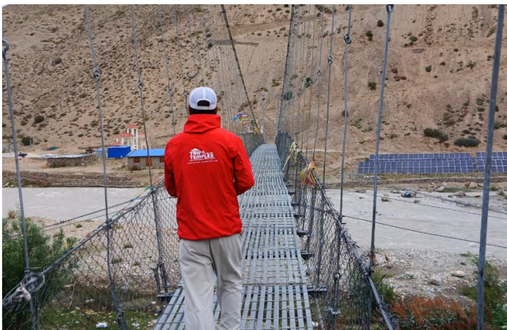
Hanging Bridge : Hilsa
